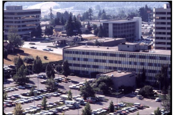
Puget Power Building on NE 4 th Street, circa 1969.
